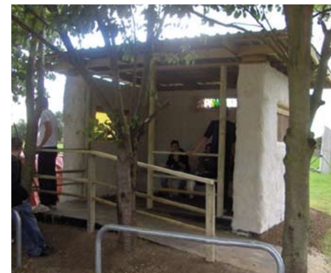
The completed eco-friendly youth shelter
