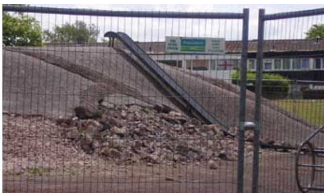
Work beginning in the park
