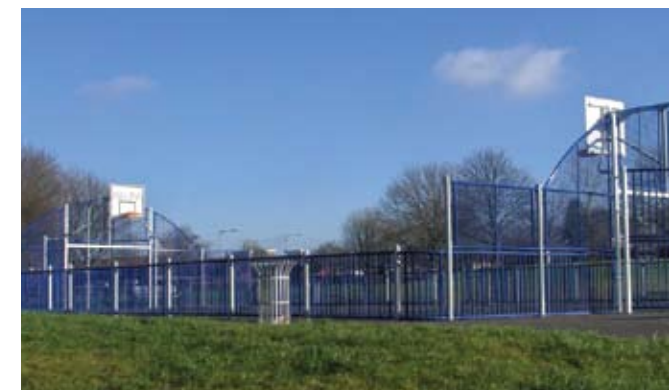
The completed Multi Use Game Arena
